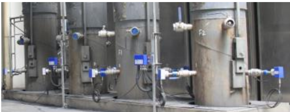
Figure 6: EUcoalflow system in a power plant, measuring the fuel mass flow in each individual coal pipe.
