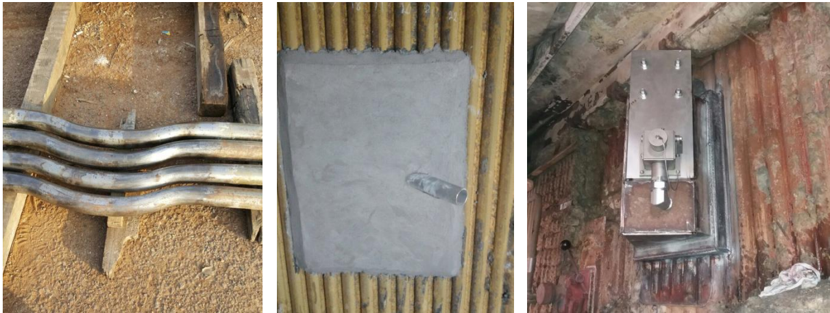
Figure 4: Tubes bending, refractory work with camera duct and camera mounting plate with EUvis air lock adapter
