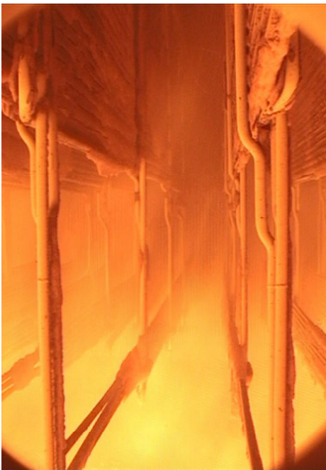
Superheater inspection
